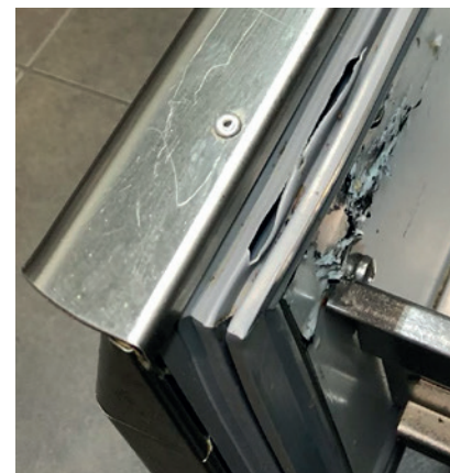
worn door seal
